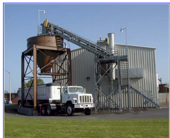
Figure 5: Solids Handling Building
